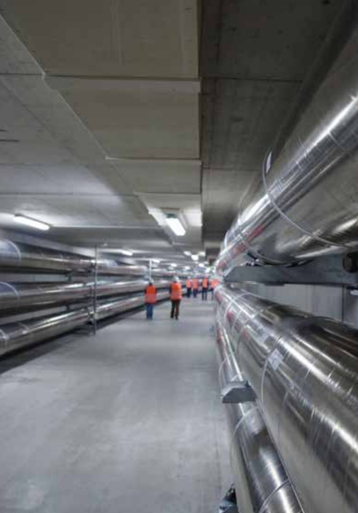
Gas-insulated lines (GIL) are an excellent alternative to overhead lines and emit almost no electromagnetic radiation.
