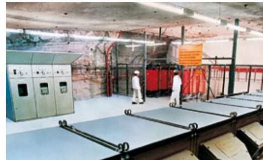
In the rolling mill directly alongside the consumer: GEAFOLE in converter operation
