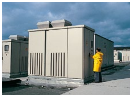
Even when space is limited: room can be found for GEA FOL transformers – even on the roof
