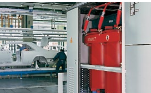
Safe: the transformer is directly beside the assembly line
