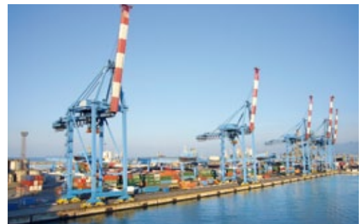
Three transformers in the crane: 6600 kVA, 37 m above the ground
