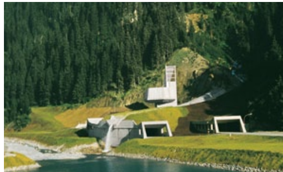
Distributed for safety: GAFOL in the Arlberg tunnel
