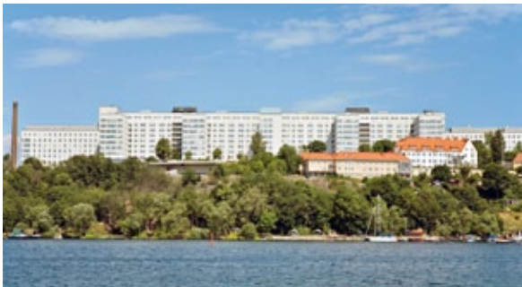
Power supply around the clock: GEA FOL in the hospital
