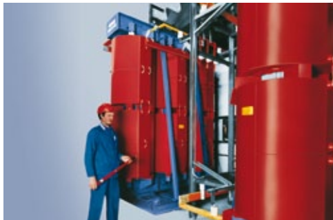
In the rolling mill directly alongside the consumer: GEAFOLE in converter operation
