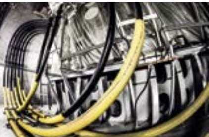
AC cable systems on offshore converter platform
