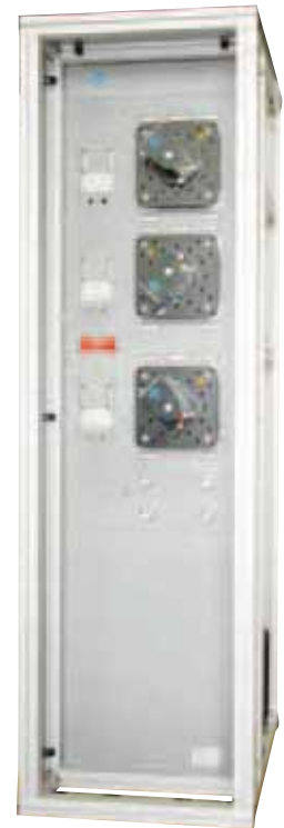
Typical design with plug in switches
