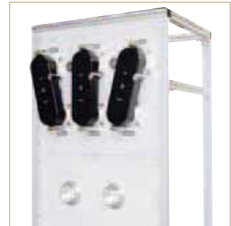
Umschaltfelder Patch Panels
