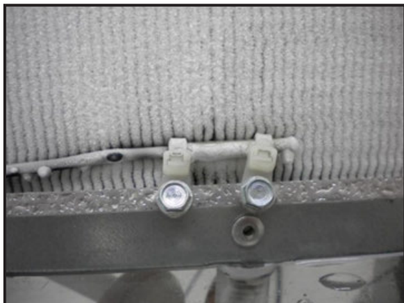
Figure 8. Iced thermistor probe on evaporator.
