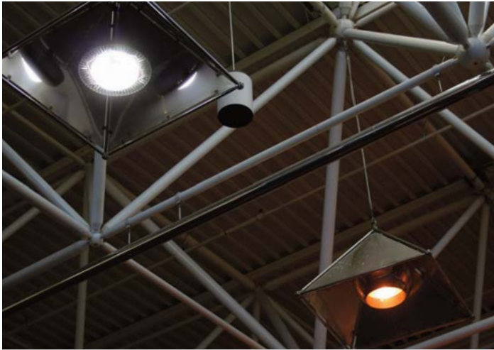
417 existing 175W Metal Halide and 150W High Pressure Sodium fixtures were replaced
