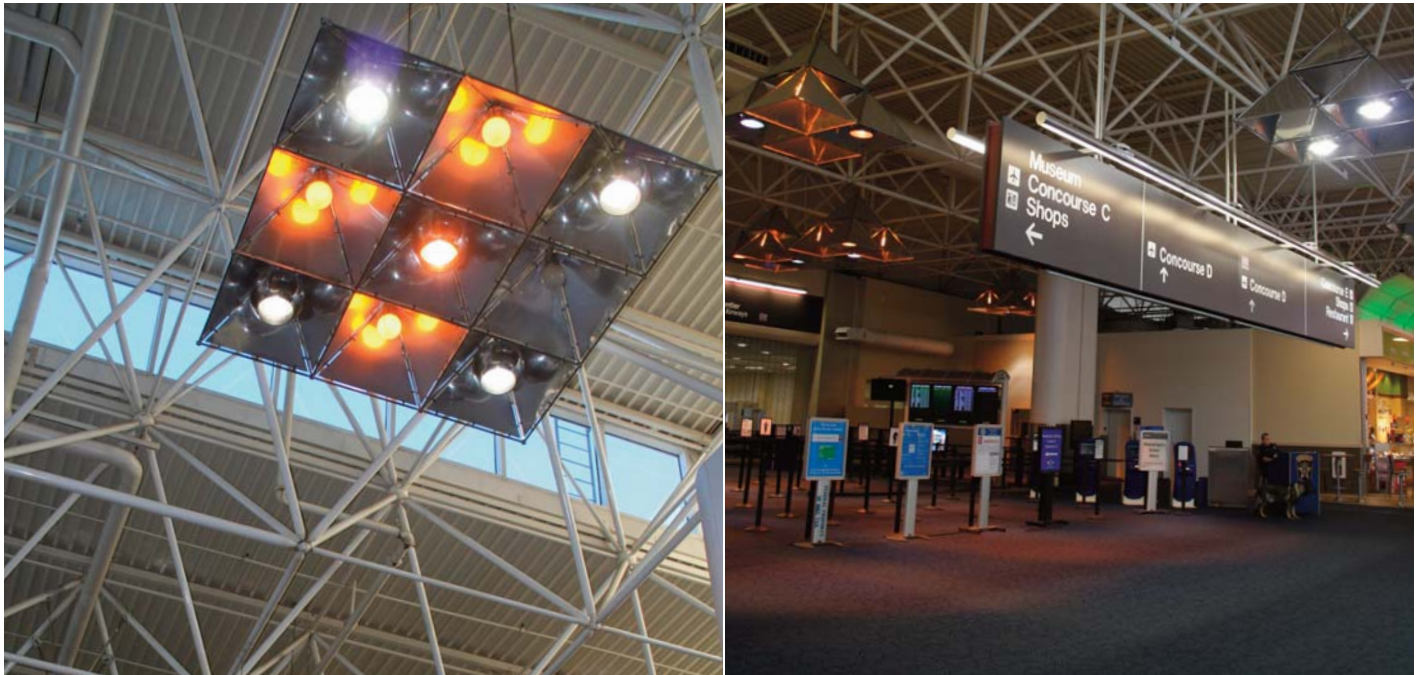
Dialight LED Low Bay fixture based on their industry leading energy and maintenance performance
