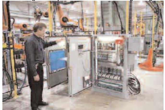
KUKA engineer, Rod Brown, at one of only two control enclosures for the entire system. Smaller remote panels are used with combination standard and safe I/O devices.
