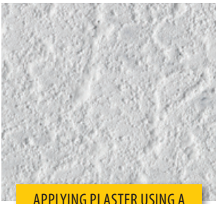
APPLYING PLASTER USING A BRUSH
