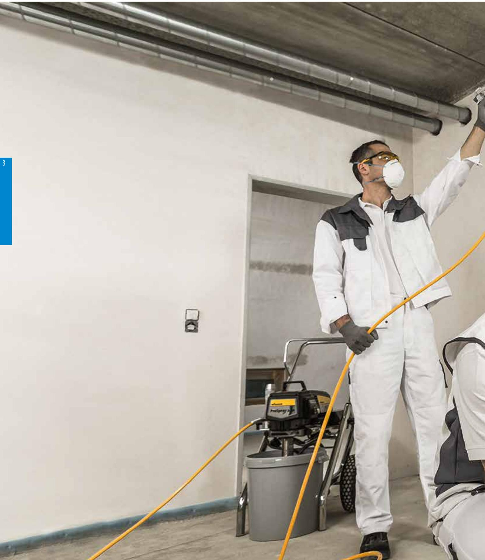
Piston pumps transport the material by means of a stroke movement in the piston. This creates high suction performance, making them ideal for highly viscous materials. Pneumatically driven piston pumps are explosion-proof and therefore suitable for use in workshops. Our hydraulic piston pumps offer even greater performance and can also be operated with petrol.
