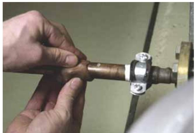
Sealing of a copper tube
