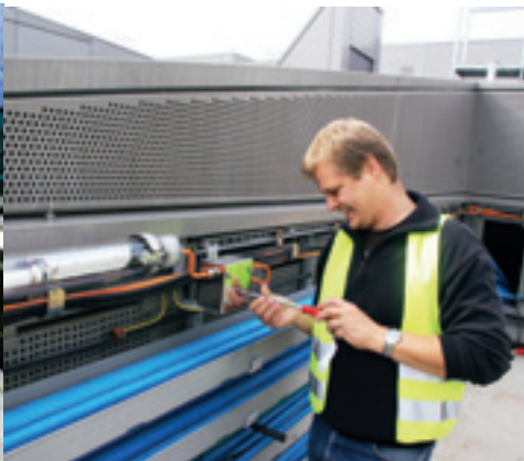
Also a part of the Viennese metro: Artwork in the Volkstheater station (left). Siegfried Schierl, project manager of infrastructure at BEA Electric (centre), tests the distribution boxes delivered by Weidmüller (right), in order to provide safe illumination along the route of the U2 line.
