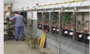
Testing Siren Cabinets
