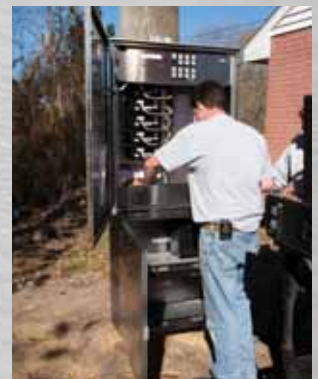
Electronic cabinet installation
