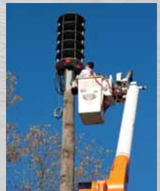
Installation of VisuAlert™ on siren
