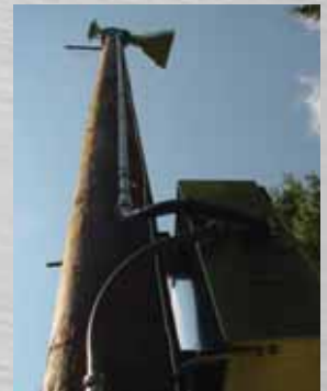
Mid-State Communications installation in Malta, NY
