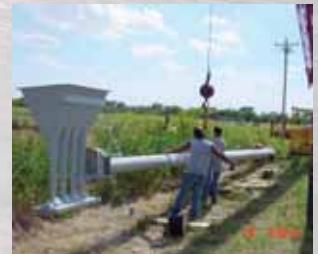
Ohio Valley Installation
