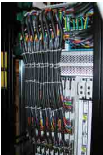
Line Card to RF Switch
