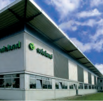
▲ Plant II, Rodezstraße in Bamberg
